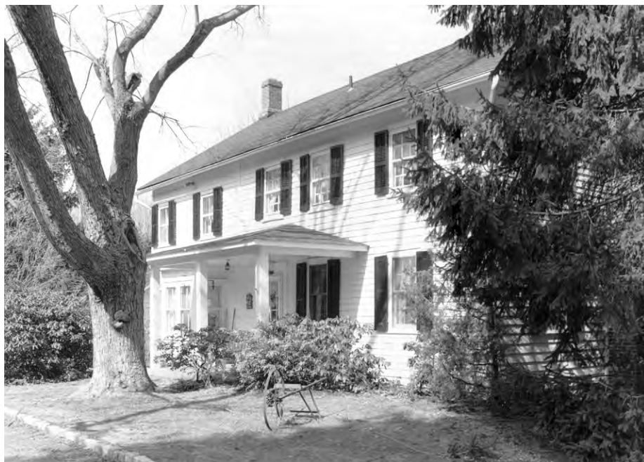
Main elevation, view northwest. 1992 photograph.
