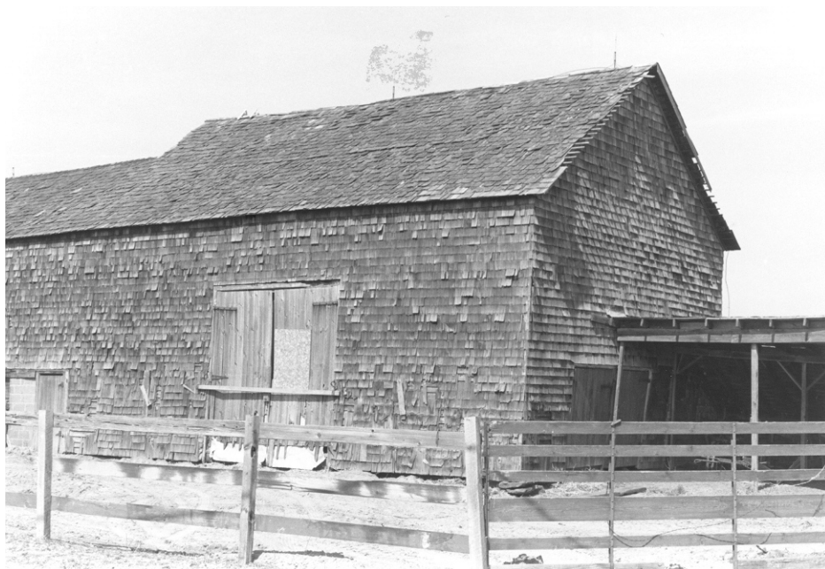
Barn C, view to northwest. 1982 photograph.
