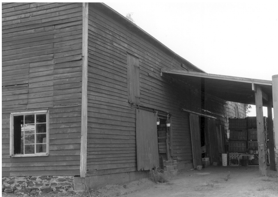
Cattle Barn A, now Packing House, view southwest. 1982 photograph.
