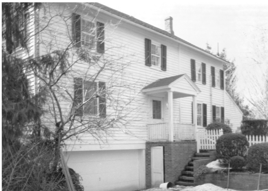
Rear elevation, view southwest. 1992 photograph.
