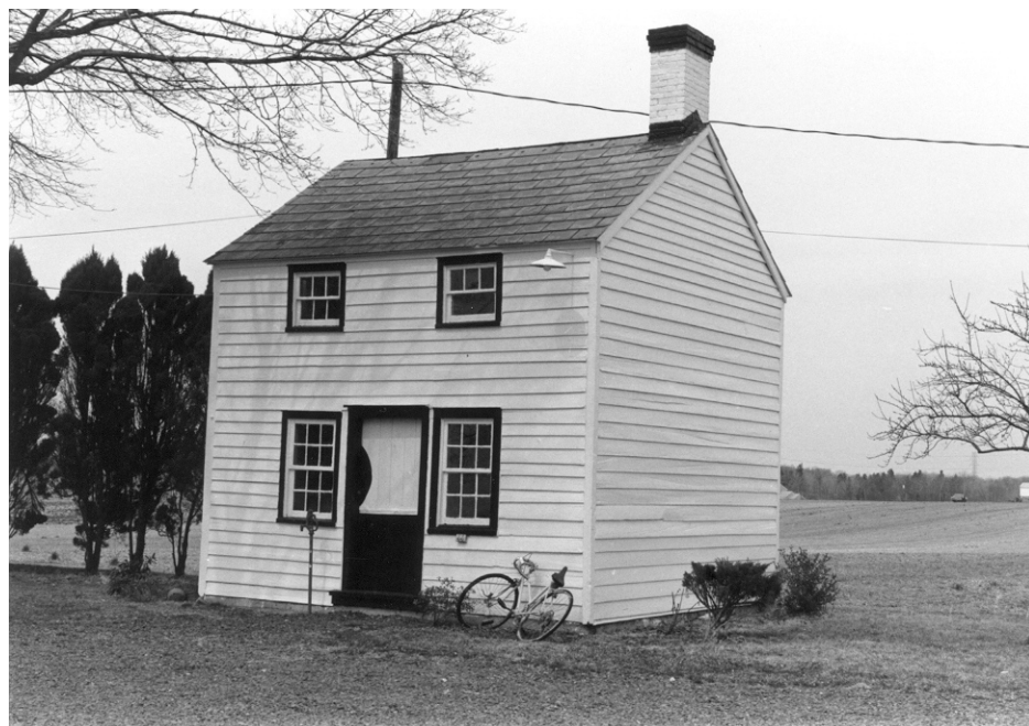
Kitchen B, view northwest. 1982 photograph.
