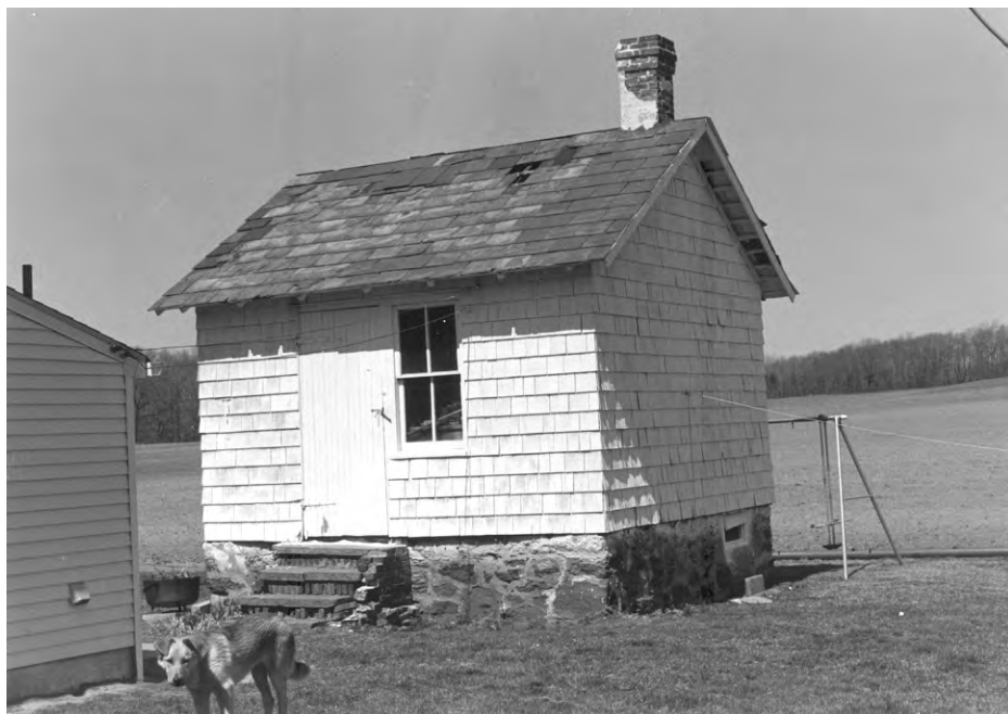
Summer Kitchen, view to northwest. 1982 photograph.
