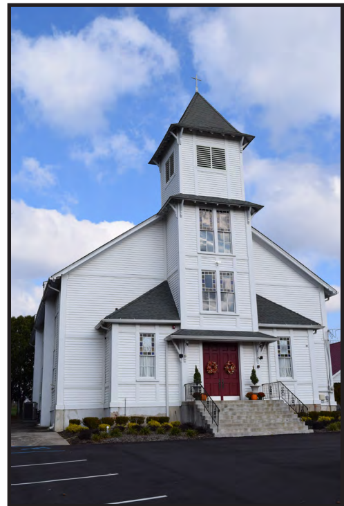
Photograph 4.26. First Presbyterian Church of Millstone, looking northeast (Photographer: Rachel Craft, November 2022; HRI Neg. #22056 D1:20).
