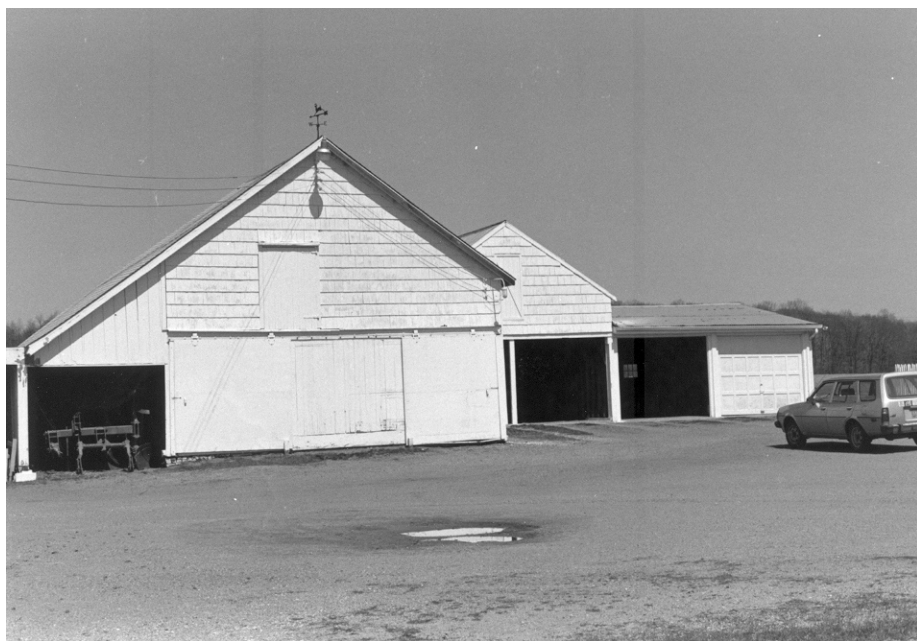
Sheds, view north. 1982 photograph.
