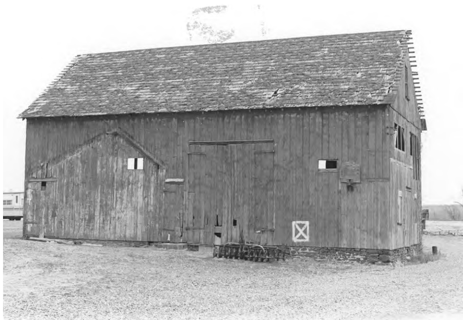
Barn C, view east. 1982 photograph.
