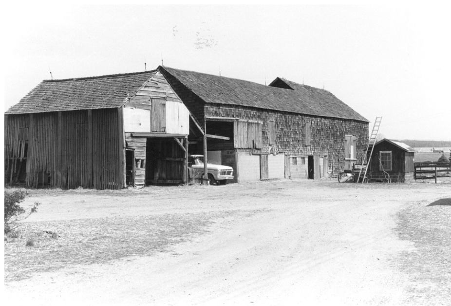
Wagon Shed B and Barn C; view to northeast. 1982 photograph.
