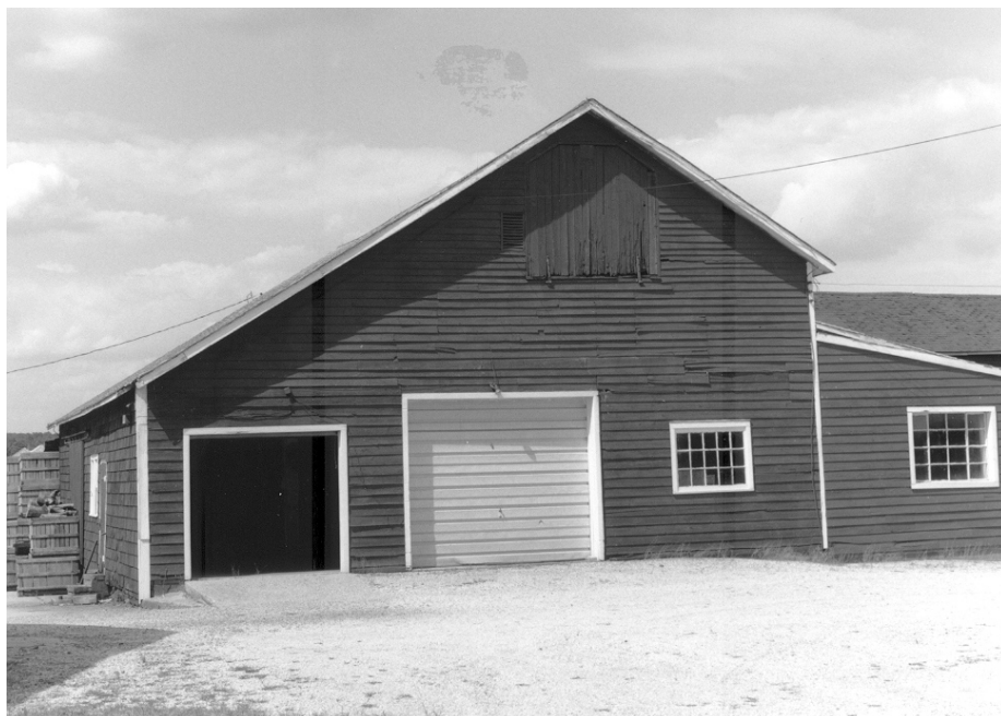
Barn C, view north. 1982 photograph.
