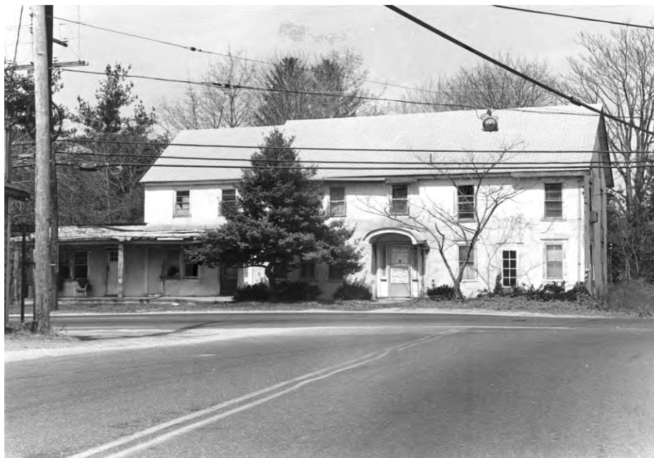
Appearance prior to rehabilitation, view northwest. 1982 photograph.
