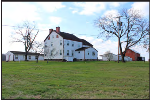
Photograph 4.32. Nathaniel Cox House and Farm, 25 Millstone Road, looking southwest (Photographer: Grace Ragosa, November 2022; HRI Neg. #22056 D2:14).
