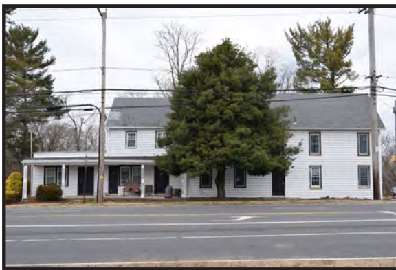
Photograph 4.22. Parker/Smithburg Hotel, 247 Monmouth Road, looking northwest (Photographer: Rachel Craft, January 2023; HRI Neg. #22056 D4:42).
