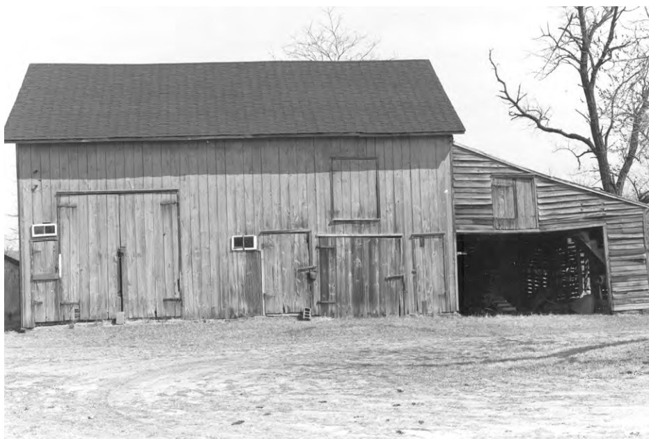
Barn, view east. 1982 photograph.
