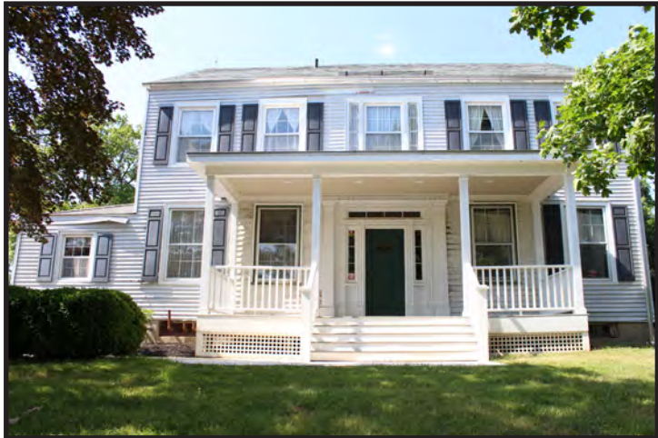
Photograph 1.1. Thomas Baird House, looking north. (Photographer: Grace Ragosa, June 2023; HRI Neg. #22056 D5:028)
