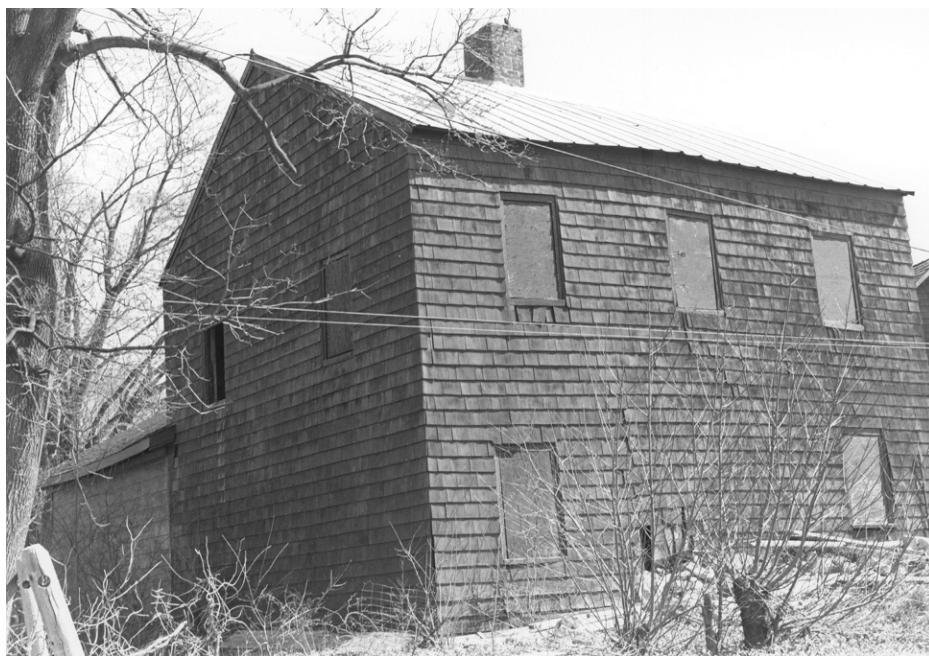
Post Office B, view east. 1982 photograph.
