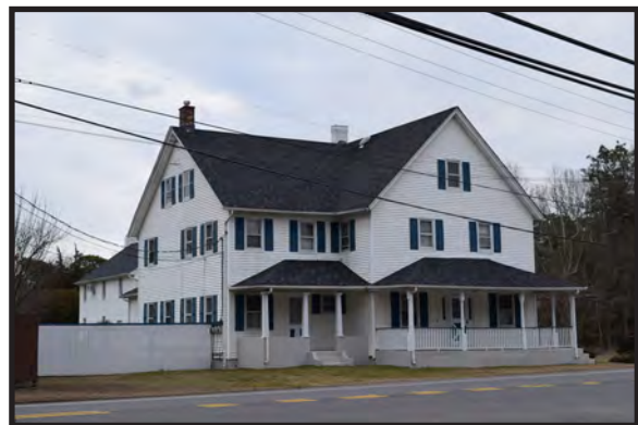
Photograph 4.23. Carr’s Tavern/Hooper General Store, 26 Trenton-Lakewood Road, looking southeast (Photographer: Rachel Craft, January 2023; HRI Neg. #22056 D4:47).
