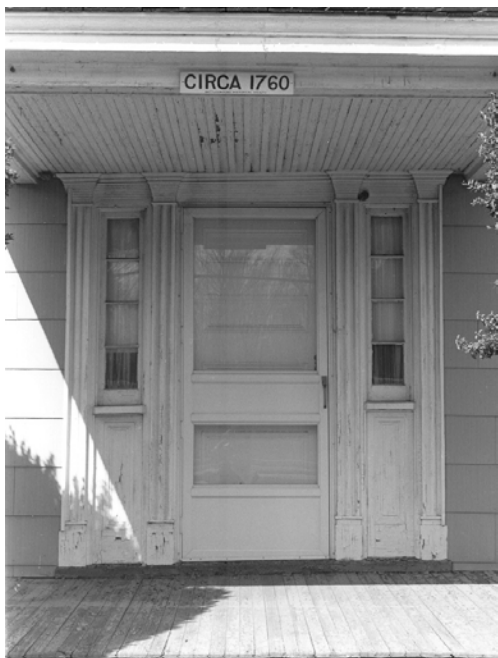
House, doorway detail. 1982 photograph.
