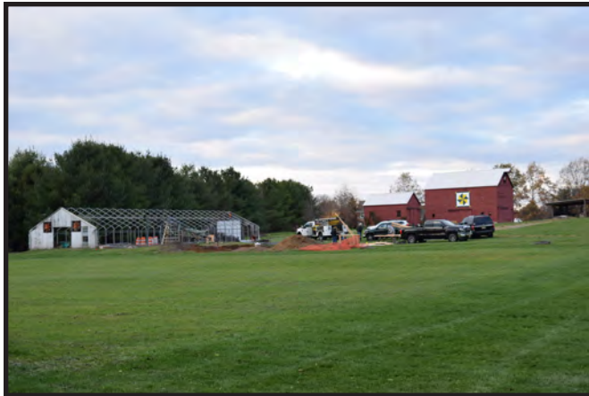
Photograph 4.11. Outbuildings at the Baird Homestead, looking northeast, with greenhouse left of view. Vehicles in mid-ground are clustered around the windmill, which was in the process of restoration when this photograph was taken (Photographer: Rachel Craft, November 2022; HRI Neg. #22056 D1:53).
